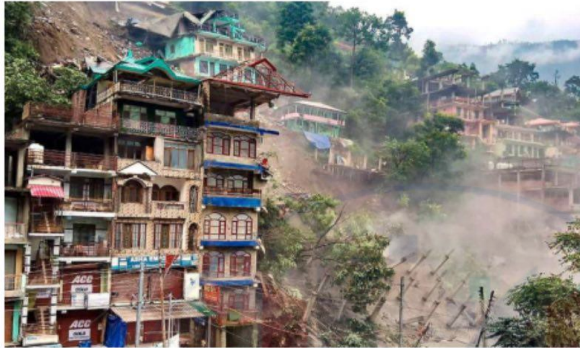
Crumbling hills: Several buildings collapsing following massive landslips at Kullu in Himachal Pradesh in August. AFP
